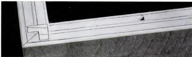
DELUXE, LOCKED-MITER CORNER , shown above, uses an L-shaped spline for accurate alignment and maximum strength. A dado head is useful but not necessary for cutting the \frac{1}{4} "-wide grooves that take the splines. If you use a regular blade, run off \frac{1}{2} "-deep kerfs to form the outer edges of each groove. In photo below, at
